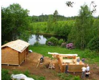
Two cabins overlooking lake
